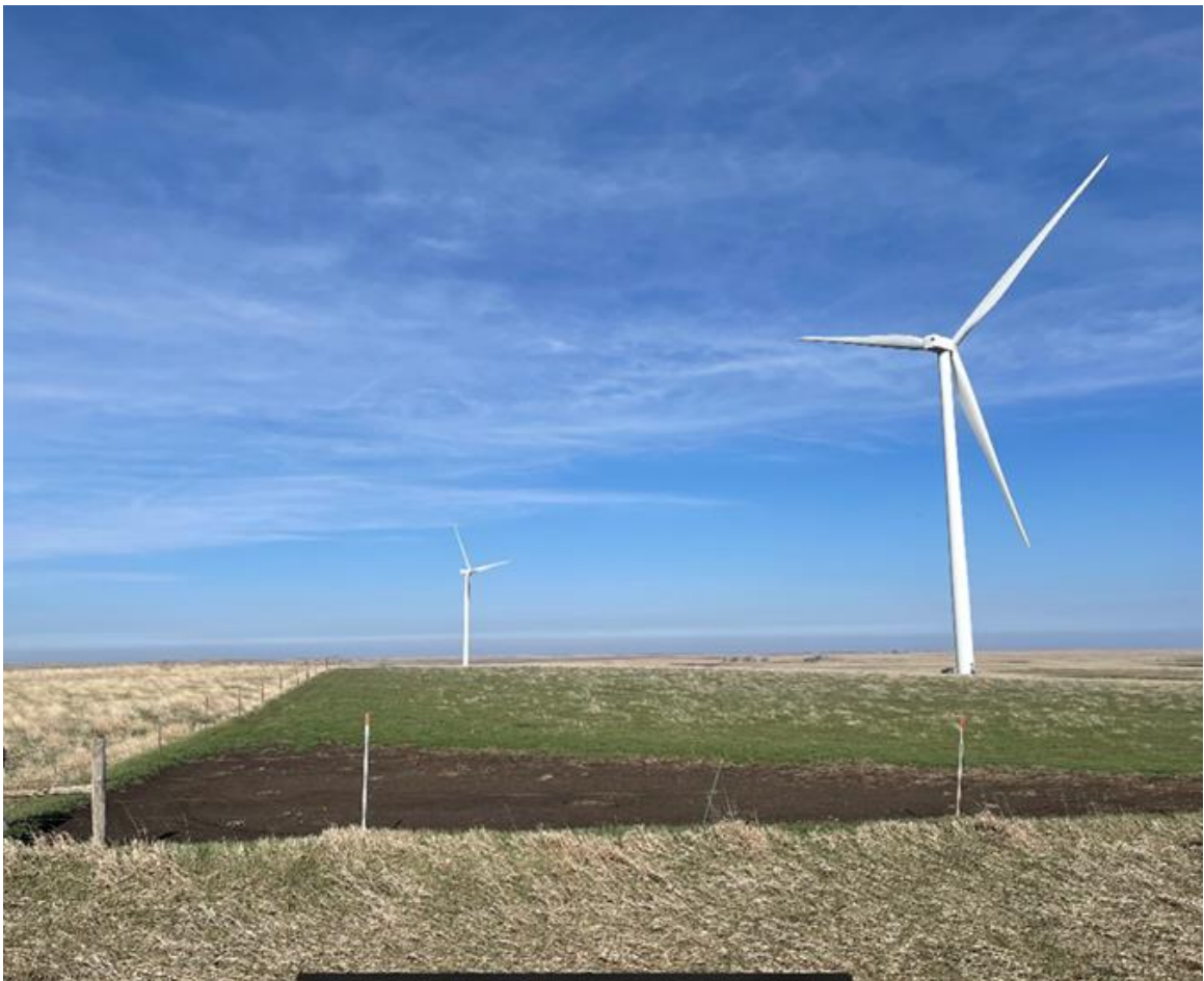
The first wind turbines on SD School and Public Lands in Hyde County
